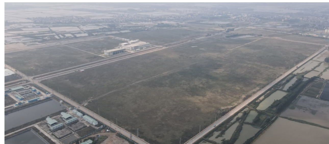
Infrastructure of Nam Son Hap Linh Industrial Park is being completed
