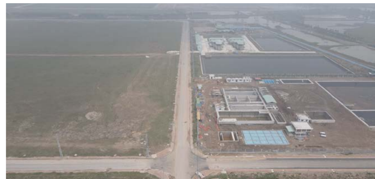
Nam Son Hap Linh IP - Bac Ninh has been put into business since 2021, there are already customers' factories under construction
